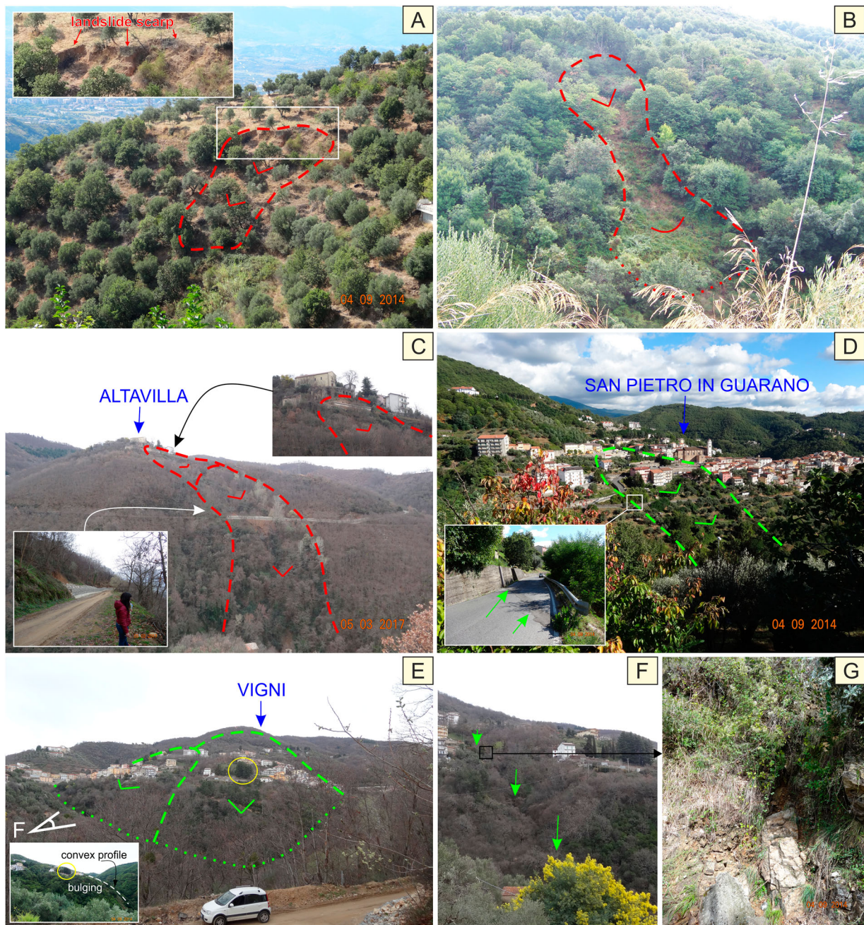
Figure 7. Types/categories of landslide affecting the study area: (A) active shallow debris slides; (B) active shallow complex landslide; (C) active medium-deep slide; (D) dormant medium-deep slide; (E) dormant rock slide (deep-seated landslide); (F) detail of the landslide flank coinciding with a NE-SW fault zone (G).
