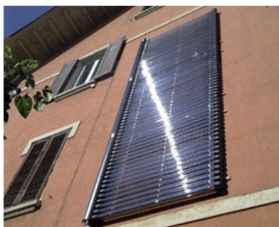
Fig. 4 Example of evacuated solar collector installation in building facade
