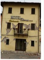
Figure 1: Damage of historic masonry walls under shear loading during earthquake October 2016 (Visso, Marche region, Italy).
