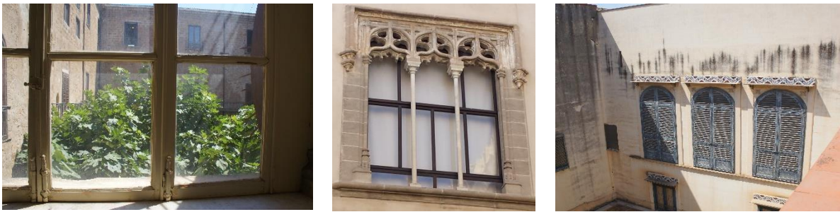
Figure 3. Few examples of windows and shadings to be preserved.
