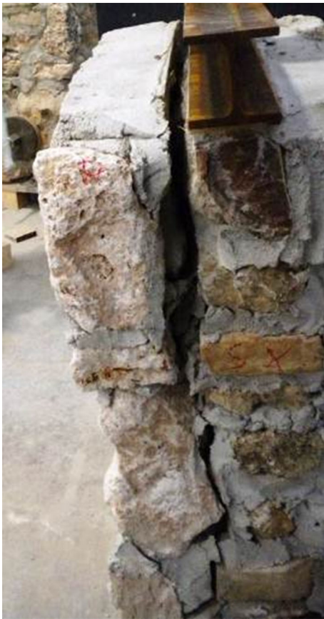
Fig. 7 Failure mode (unreinforced panel)
