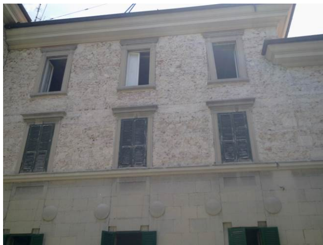
Fig. 8. Detail of bricks layout on the west wall, third floor.
