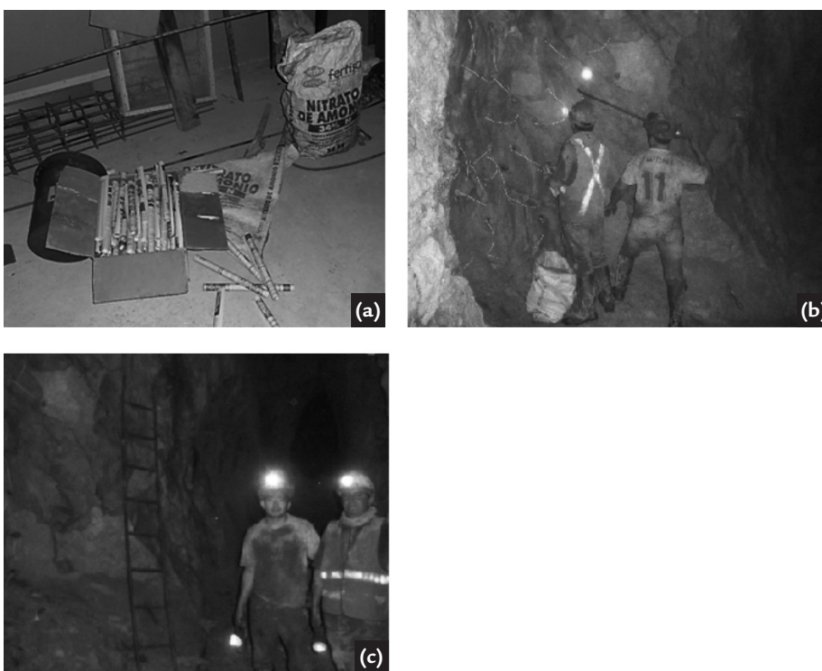
Figure 2 (a) Ammonium Nitrate bag and empty newspaper cartridges; (b) charging of a blast and (c) operators ready to ignite the fuses. In b/w for a better resolution of the pictures taken underground.
