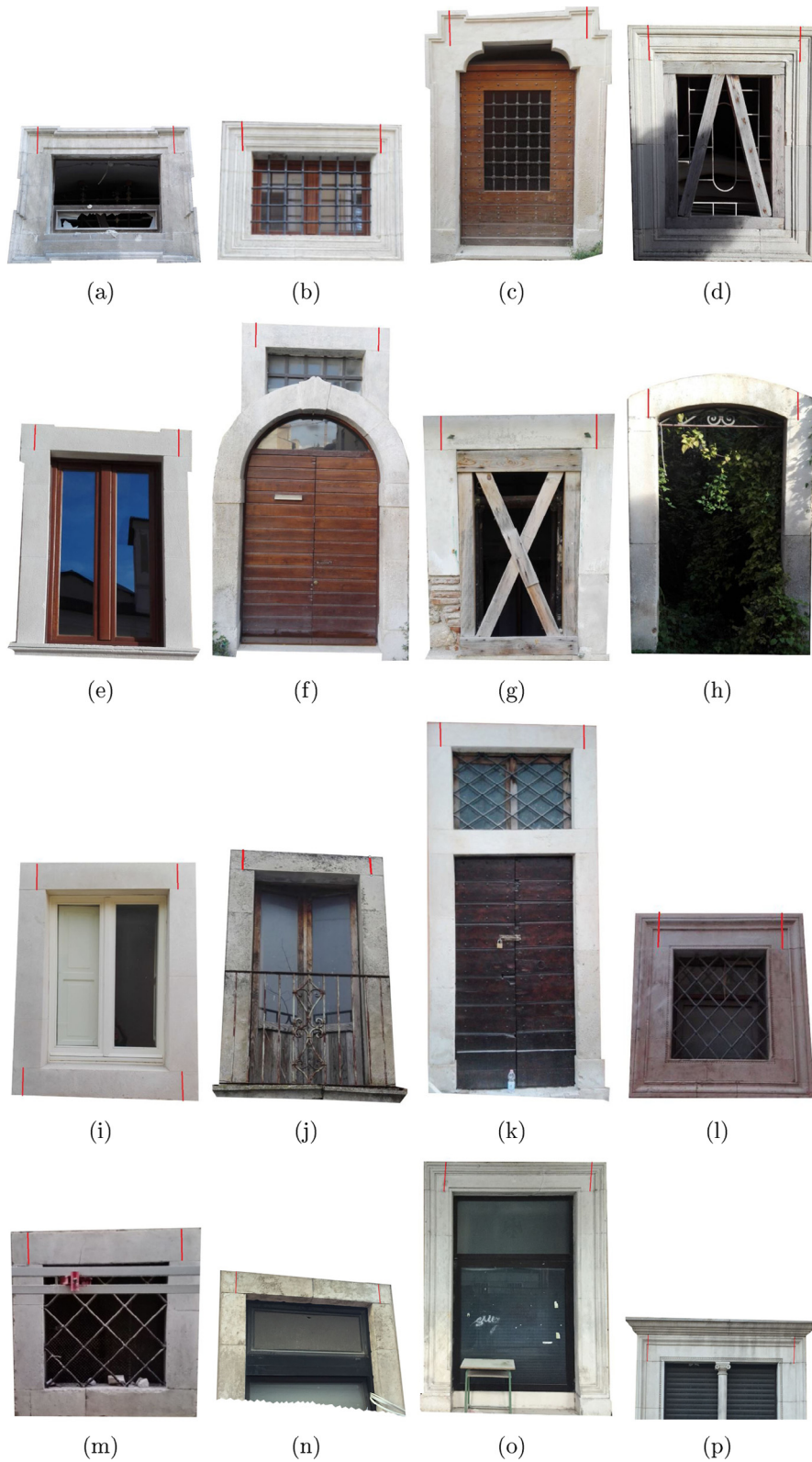
Fig. 2. Examples of the PT architrave. The red lines highlight the dis-articulation of the architrave into three elements, the block spanning the opening and the two lateral pieces.
