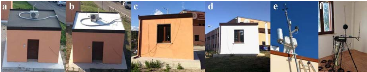
Fig. 1. Case study building: (a, b) roof configurations; (c, d) façade configurations; (e) outdoor and (f) indoor microclimate monitoring setup.
