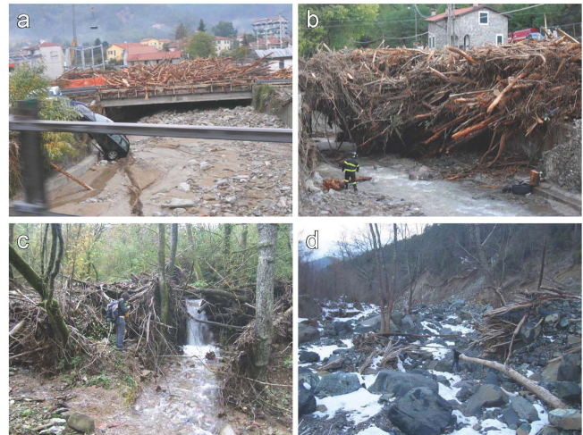
Figure 1. (a) LW clogging in the Magra river catchment after the 2011 flash flood, upstream view of a bridge in the town of Brugnato. Note also the evident sediment deposition below the bridge; (b) downstream view of a huge wood jam trapped by a bridge in the village of Pignone; source: Autorità di Bacino Interregionale del Fiume Magra and Provincia della Spezia. (c) A LW jam anchored on remaining vegetation, it retained sediment upstream; (d) LW jam deposits anchored by the remaining vegetation.
