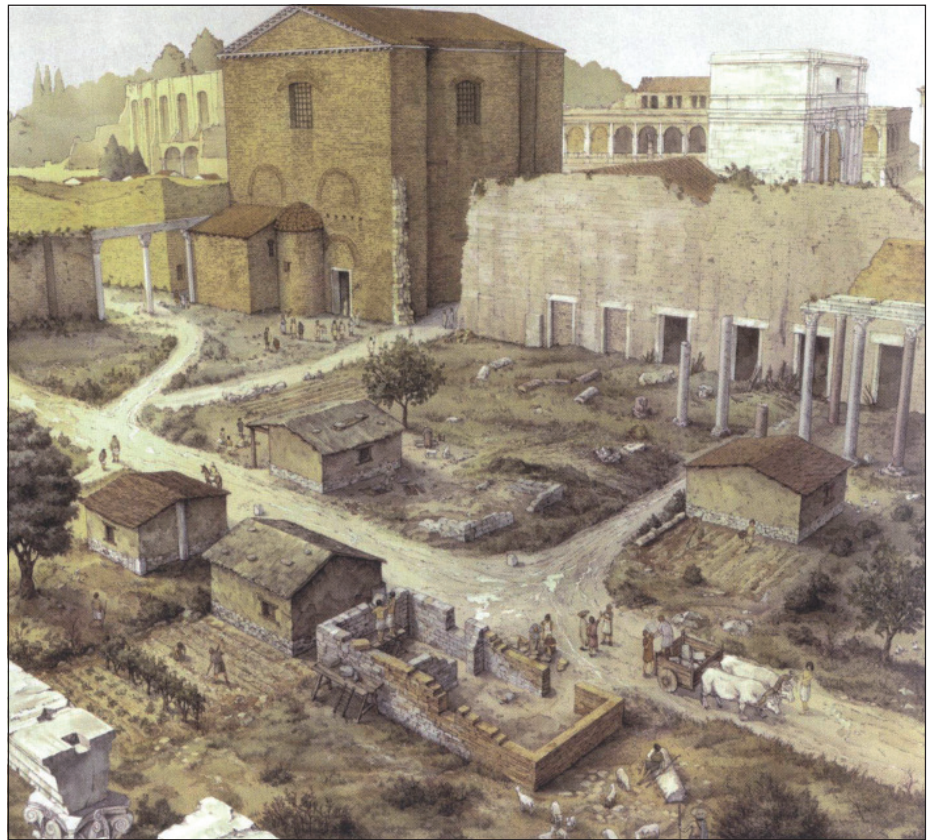
Fig. 7. Two-storey 9th century houses from Nerva's Forum, Rome (from Brogiolo 2011, p. 176, fig. 82)
