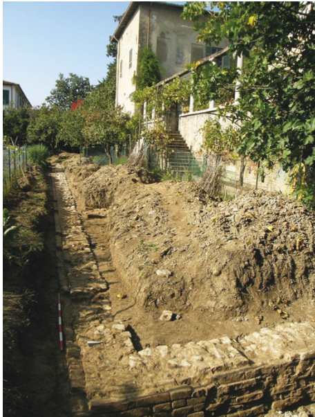
FIGURE 16: C-zone: a nearly east-westward view of the foundations of the fourth wing of the Castle of Zena found in correspondence of the inner sequence of nuclei at right angle in the geoelectrical tomography of Figure 11.
