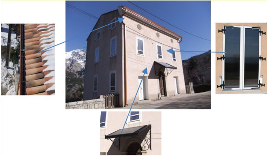
Fig. 57.7 Historical building with integrated solar systems
