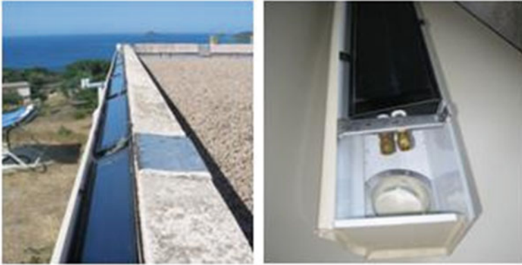
Fig. 57.6 Patented solar collector H2OSS
