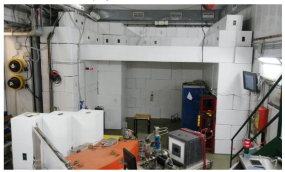
**Figure 2.10:** During the July-September 2015 shutdown the concrete block shielding of the BTF experimental hall has been dismounted and reinstalled in an improved configuration, adding a concrete ceiling (50 cm concrete).
