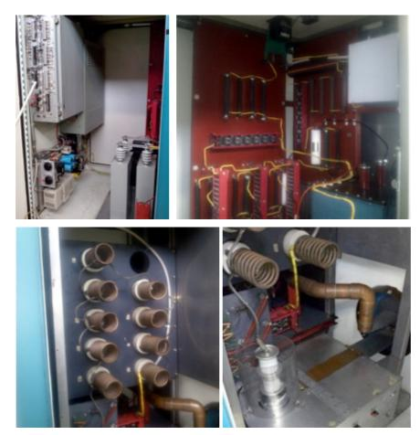
**Figure 3.3:** The SCR rectifier, the core bias and filament power supplies are placed inside one door of the modulator racks (top left), together with the diode arrays, the large charge capacitor and filters of the charging circuit (top right). In the other rack door: the 9 LC cells PFN (bottom left), the Hydrogen gas thyratron and the conductor towards the pulse transformer (bottom right).
