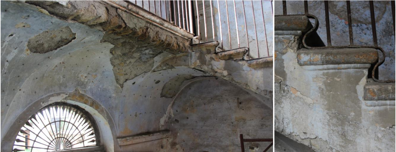
Figure 10. Details of the access staircase to the main floor.
