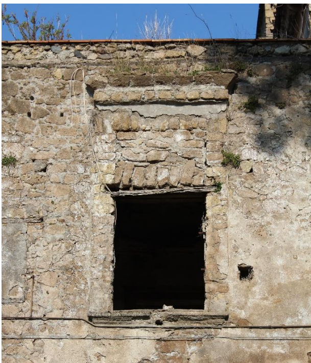
Figure 9. Detail of the south-east.
