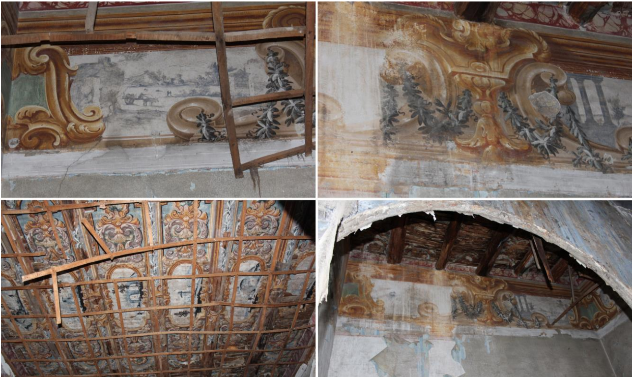
Figure 11. Details of the 18th-century parietal decorations and 'incartate' that covered the wooden floors of the main floor, later covered by ceilings as part of 19th-century modernization.
