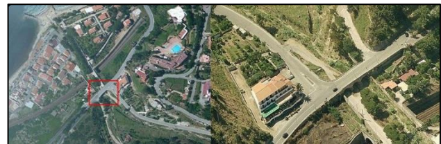
Figure 5. Bridge framing in Villa San Giovanni
