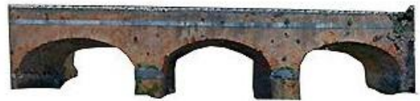
Figure 14. Texture of the Villa San Giovanni Bridge by Laser Scanner
