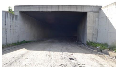
Figure 4. Detail of the tunnel entrance
