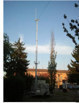
Figure 8: Temporary base station in Camposanto
