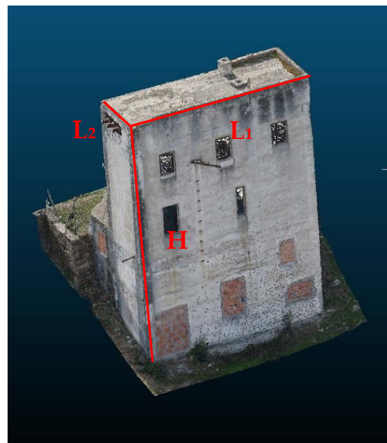
Figure 5: The measurements taken on the building
