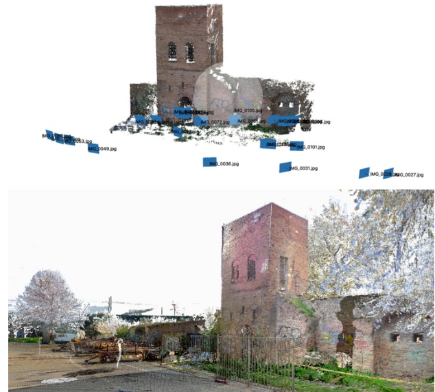
Figure 12. Above, one of the work chunks obtained by photomodelling, below a partial view of the point cloud obtained by laser scans
