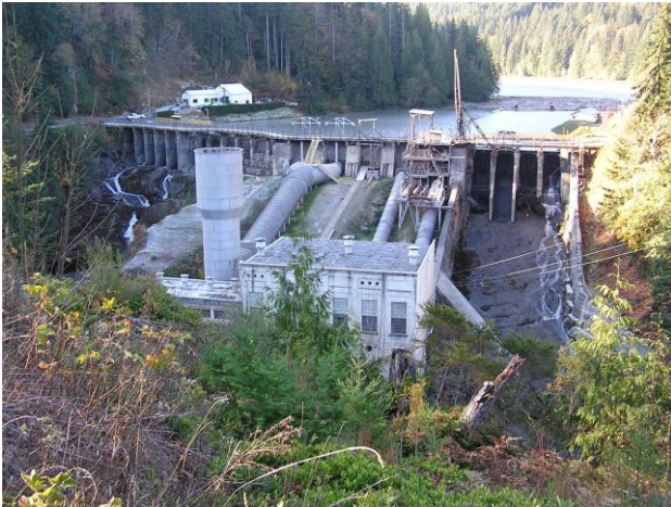
Figure 3. Elwha Dam before removal (Ward, 2005)
