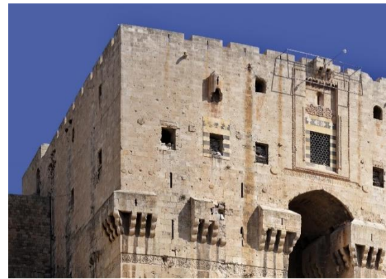
Figure 6: Entrance tower of the Citadel.
