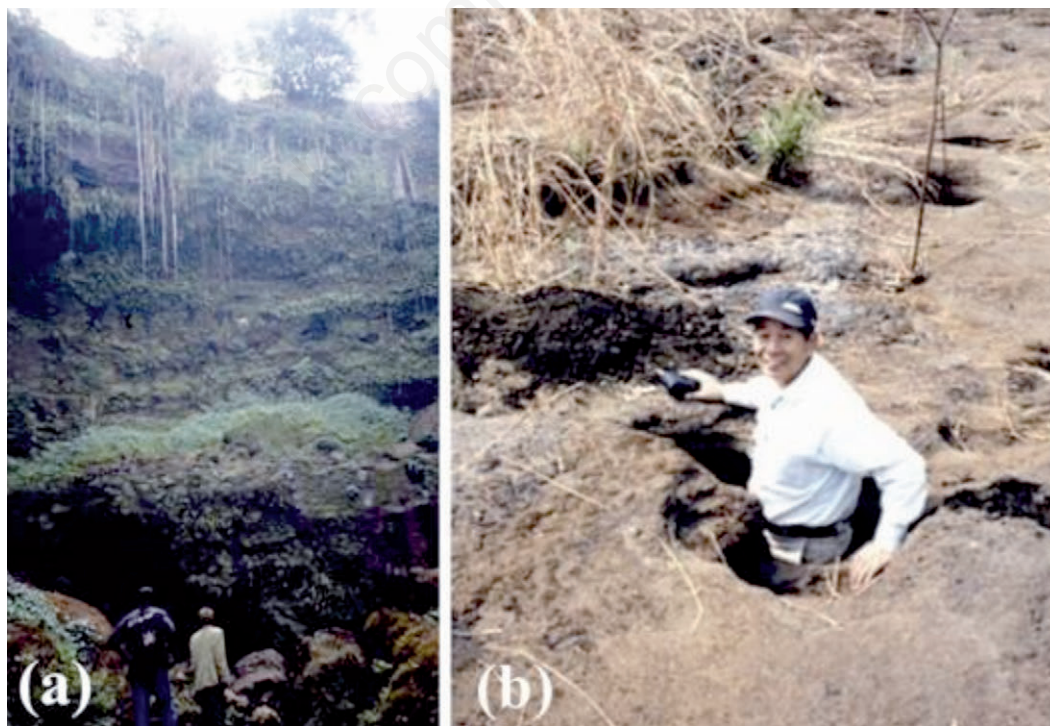
Fig. 3. a) The north wall of the Nyos dam, composed of pyroclastic rocks; note the people for scale. b) M. Kusakabe inside a pothole on top of the Nyos dam, demonstrating the mechanical weakening of the dam structure.
