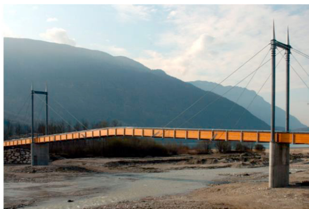
Fig. 1. Lateral view of the Tesa footbridge.
