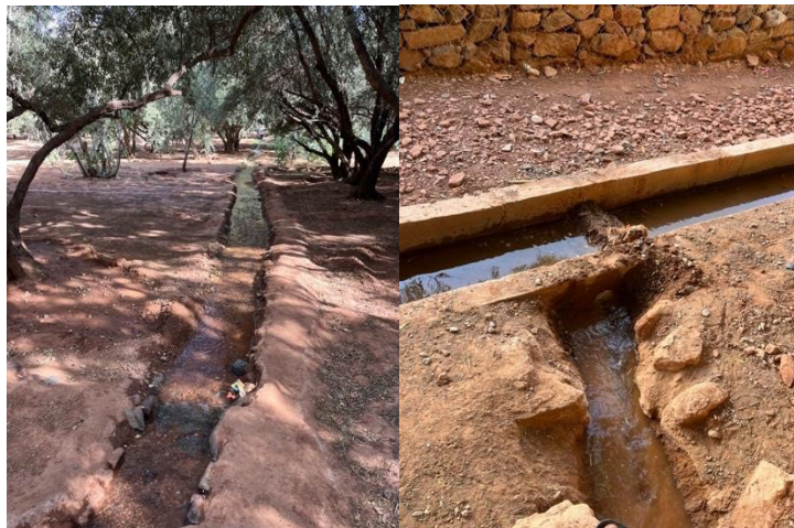
The sub-canal travelling away from the saqiya and the transition from saqiya to sub-canal. 3 November 2022.
