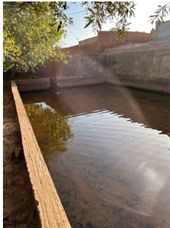
First reservoir filling with water. 3 November 2022.
