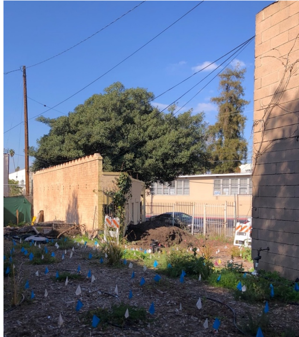
Figure 3. (Left) Image of soil remediation testing site and restaurant structure to be demolished. Taken January 28, 2023.
