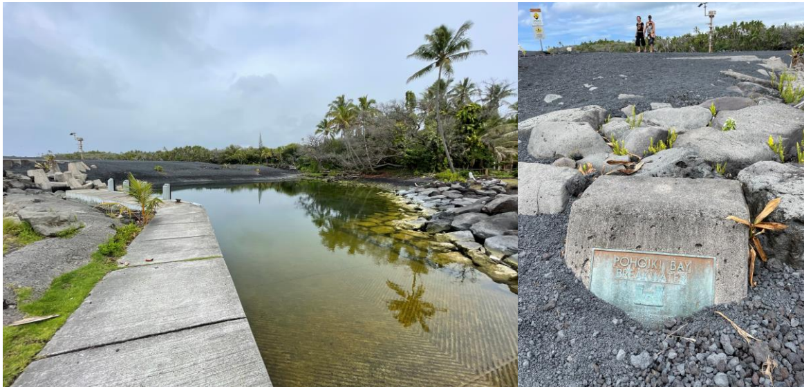
Figure 19. The Pohoiki boat ramp blocked by the lava, left. Former Pohoiki Bay breakwater, right (Shridhar 2022).
