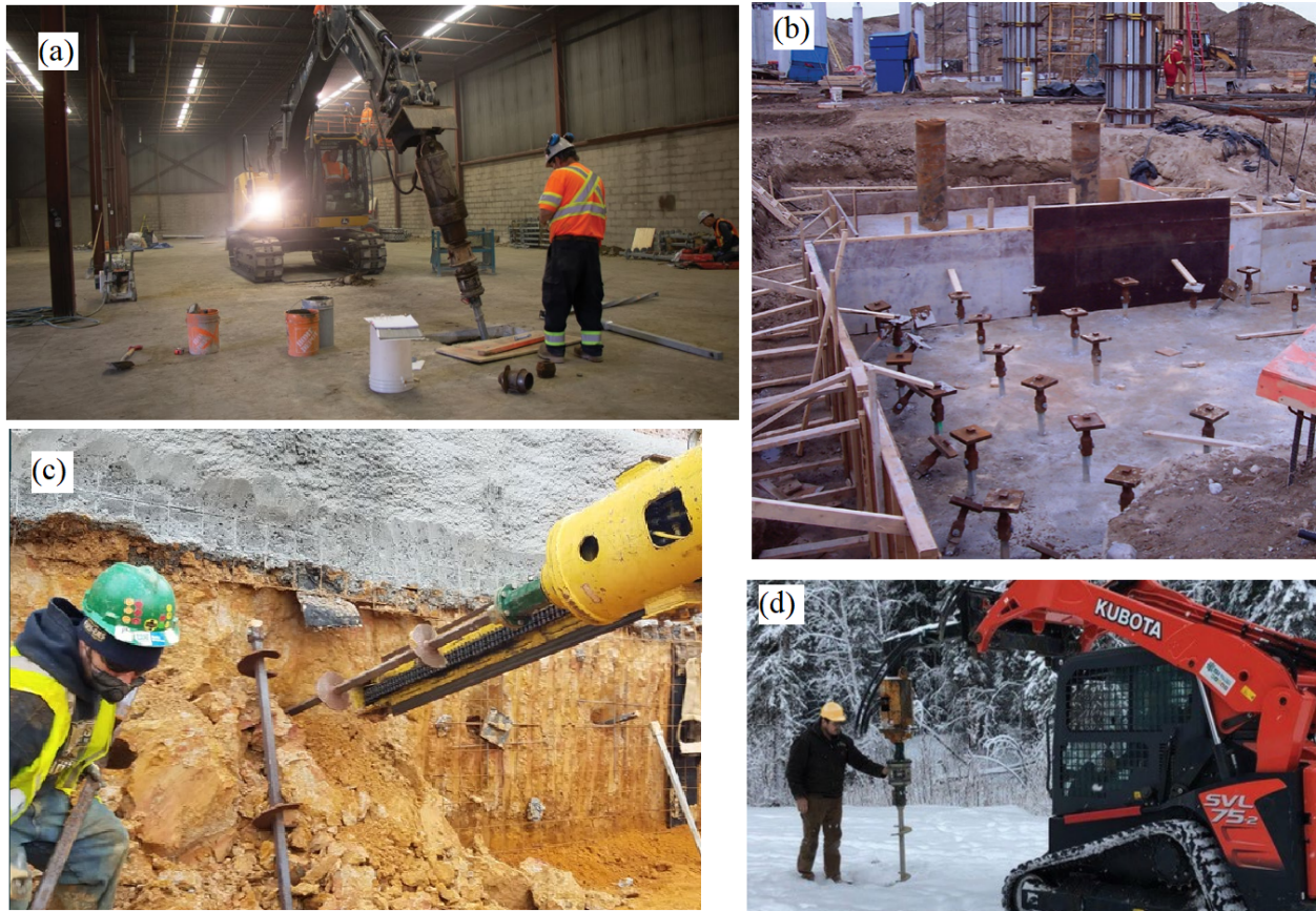
Figure 2.2: Helical piles usage: (a) installed inside existing buildings; (b) pile foundation; (c) retaining wall tie-back anchor; (d) installed in extreme weather (Courtesy of Hubbell Power Systems Inc.).
