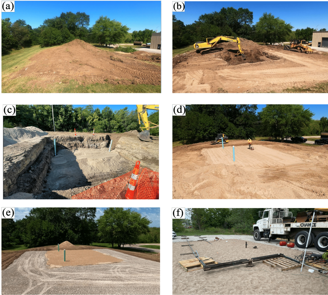
Figure 3.9: Sand test pit construction sequence.
