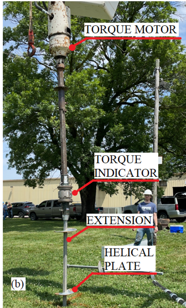
Figure 2.1: Helical pile: (a) basic components and (b) installation at Hubbell Power Systems Inc. Centralia, MO.
