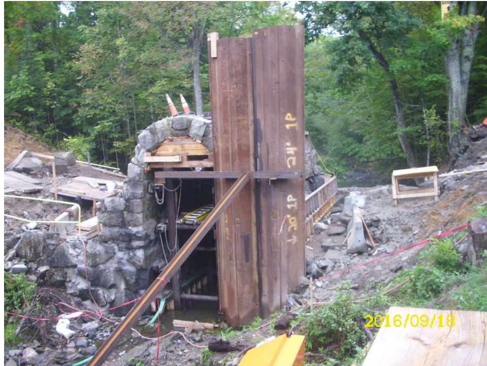
Figure 13. Stackpole Bridge during rehabilitation (Friends of Stackpole Bridge)
