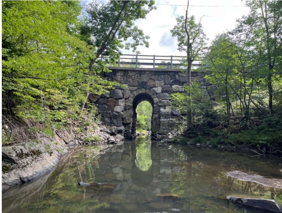
Figure 10. Stackpole Bridge after rehabilitation
