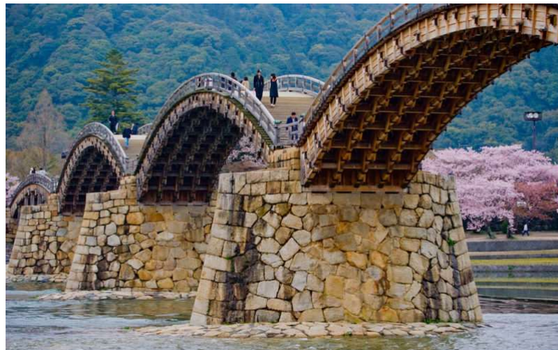
Figure 7. Kintaikyo Bridge, Iwakuni City, Japan (GaijinPot Travel)
