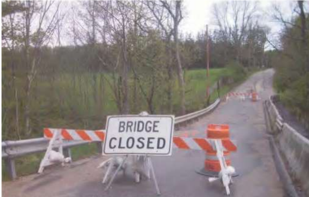
Figure 12. Stackpole Bridge when it was closed in 2013 (Maine Preservation)
