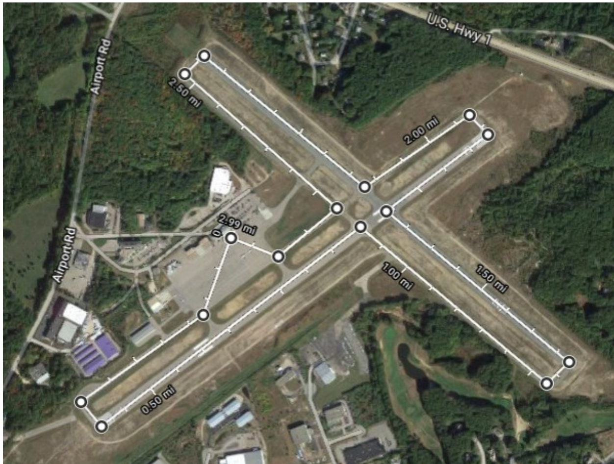
Figure 142: Inspection Route of the runway and taxiway lights
