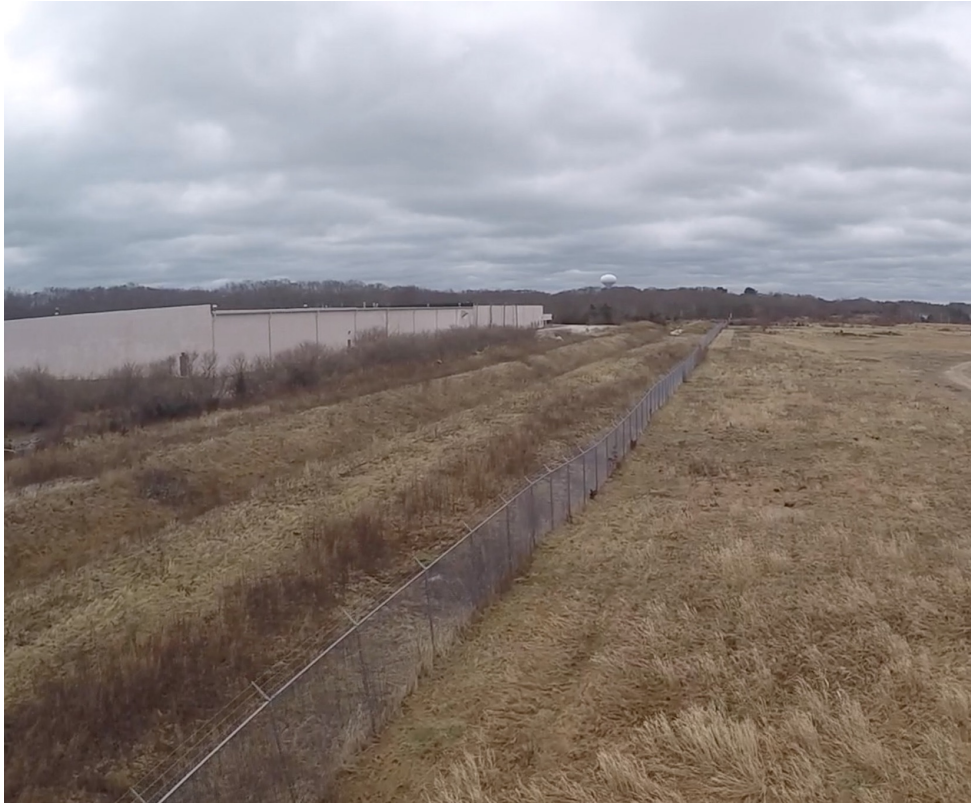
(a) Fence in perimeter inspection
