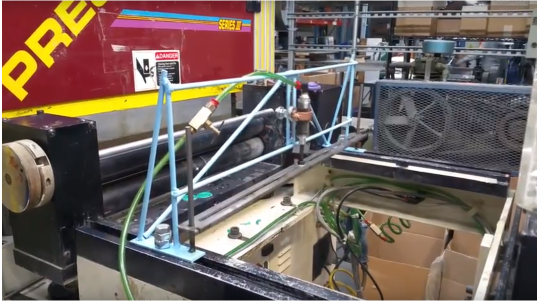
Figure 19: Installed knockout frame being tested.
