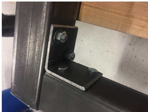
Figure 13.1: BOLTS AND BRACKETS
