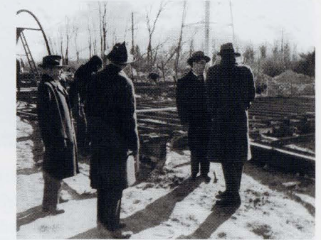
OVERSEEING ERECTION OF QUONSET HUTS, CA. 1946
