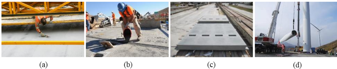
Figure 3.3: Structural applications of UHPC; (a) overlay (UT) [10], (b) UHPC joints (OR) [10], (c) waffle deck panels (NE) [63], [64] and (d) wind turbine towers(IA) [62], [65]
