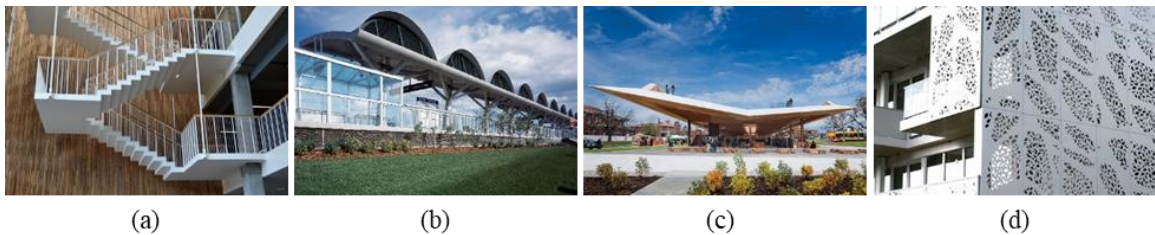
Figure 3.4: Architectural applications of UHPC; (a) Staircases (DK), (b) Sunshade (CA), (c) Gateway Pavilion (US) and (d) Facade Cladding Panels (Fr) [68]
