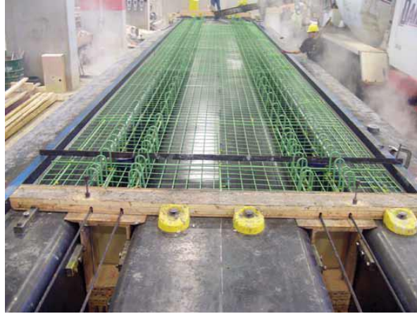
Figure 2.11: NEXT beam section at Dailey Precast plant, Shaftsbury, Vermont [5]
