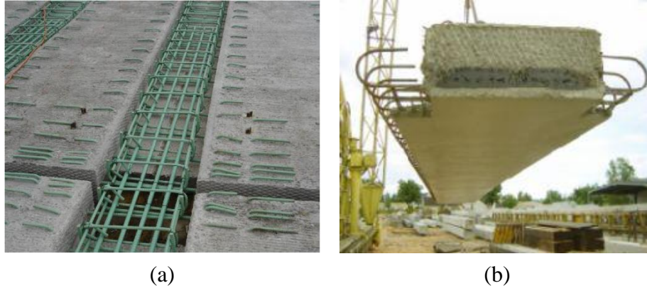
Figure 2.30: Additional reinforcement required in (a) transverse direction [59] and (b) extending from side of members [60]
