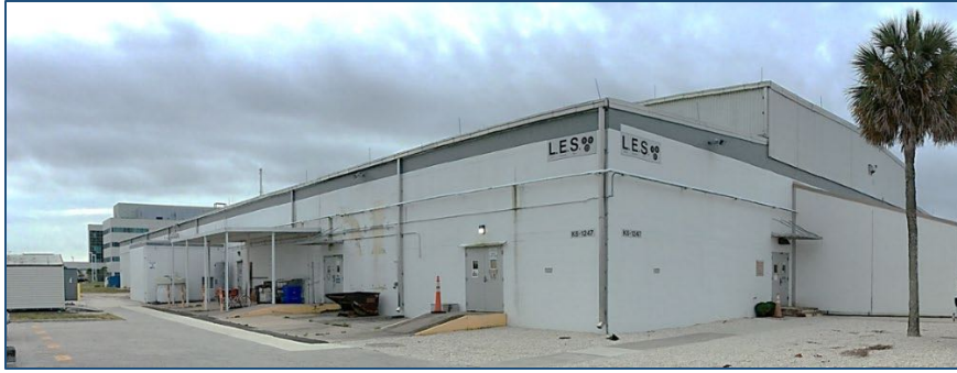
Figure 28: NASA KSC LES machine shop used for the application of chromate conversion coating onto Al2219 substrates.
