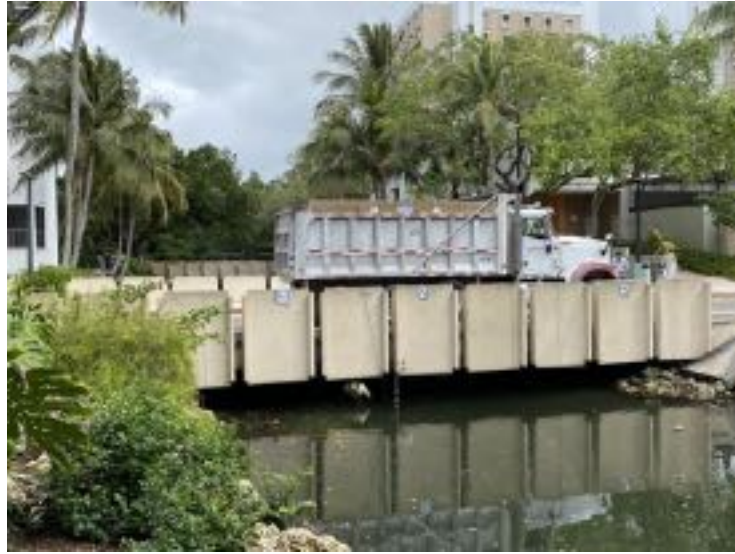
Figure 1-8. Non-destructive bridge load testing for the assessment of damaged bridges.
