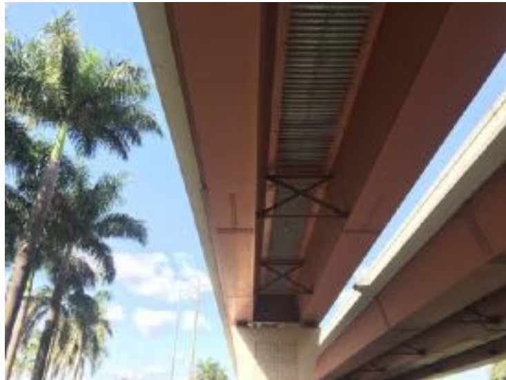
Figure 1-3. Twin steel box girder bridge classified as fracture critical.
