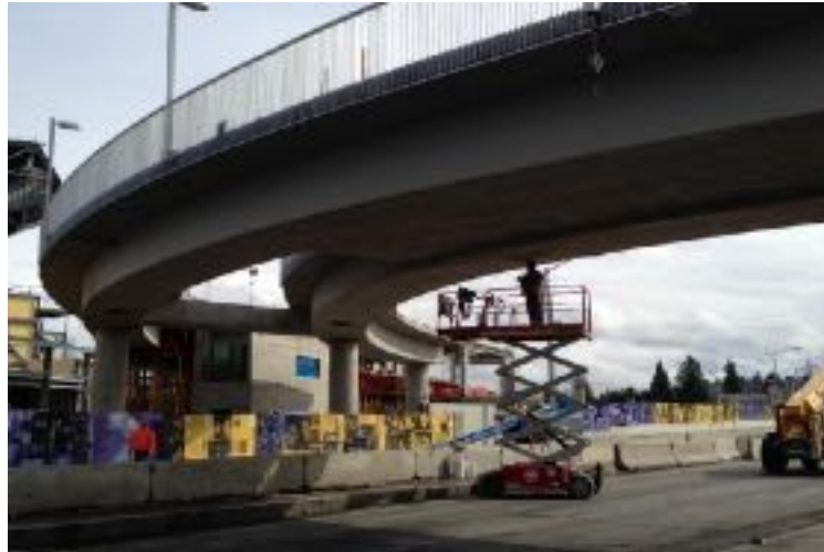
Figure 1-2. In-depth bridge inspection near mid-span over a busy roadway.
