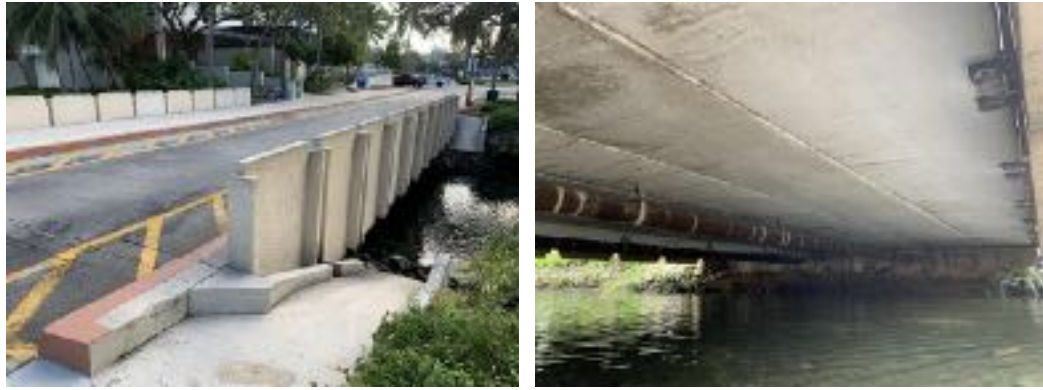
Figure 3-1. College Drive Bridge. (a) Top view; (b) Bottom view.
