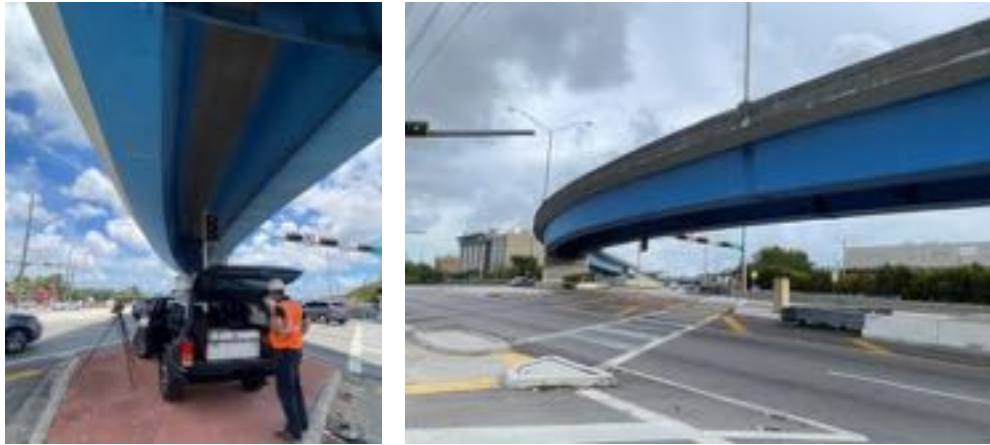
Figure 2-88. Field test using a laser vibrometer on the three-span continuous bridge.
