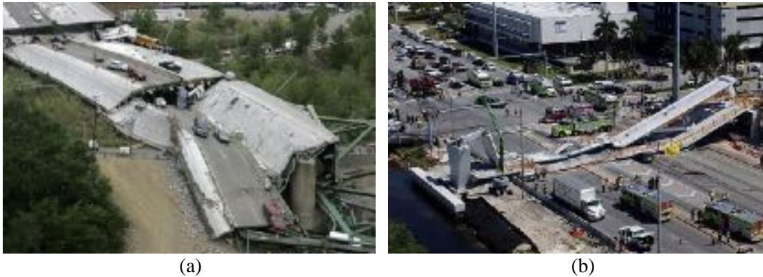
Figure 1-1. Bridge collapse;(a) I-35 W bridge over Mississippi River in 2007 [2], (b) FIU pedestrian bridge in 2018.
