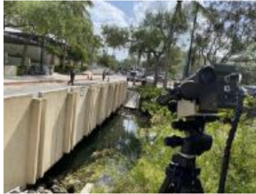
Figure 3-14. Laser vibrometer used for recording bridge vibration during the dynamic load test.
