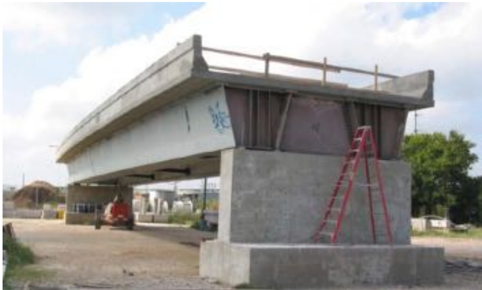
Figure 2-27. The University of Texas twin steel box girder bridge.
