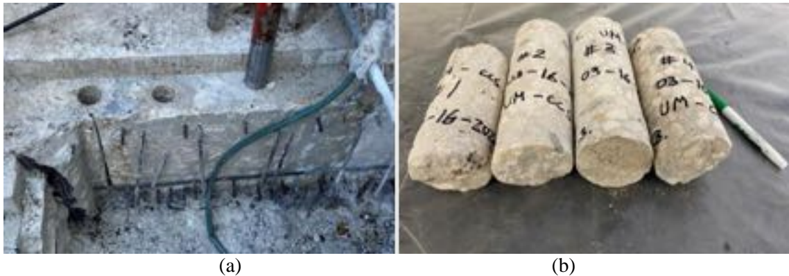
Figure 3-4. Extraction of concrete cores from the end of the precast concrete slab; (a) Sample extraction; (b) Core samples.
