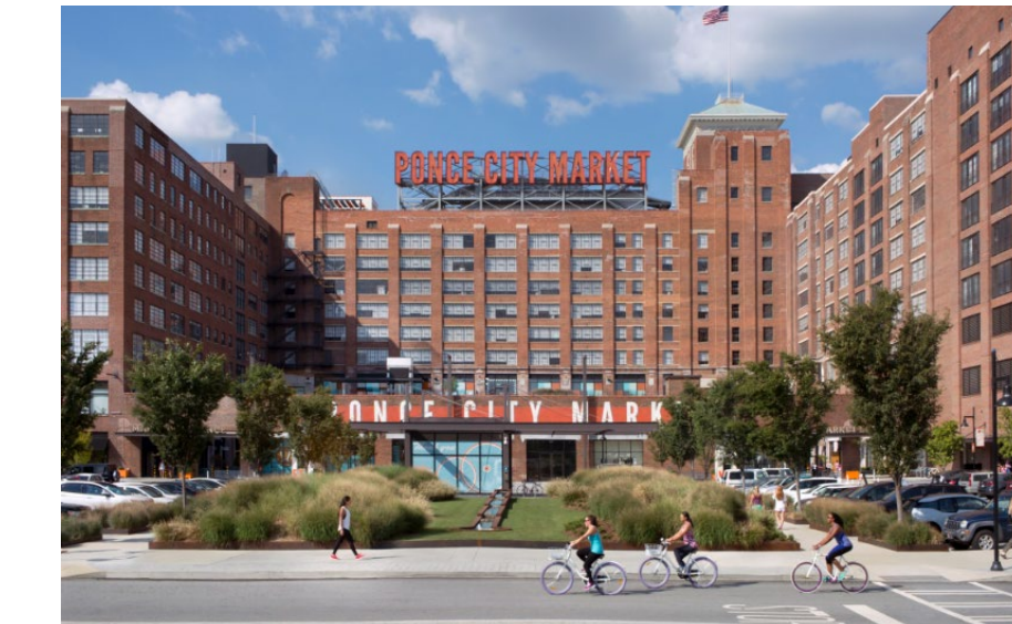
Main entry (vehicular)
