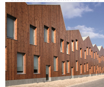
Figure 2.51 - School Center Mouriz http://mrg.pt/en/portfolio/go/mrg-construction-ebj--ji-mouriz--mouriz
