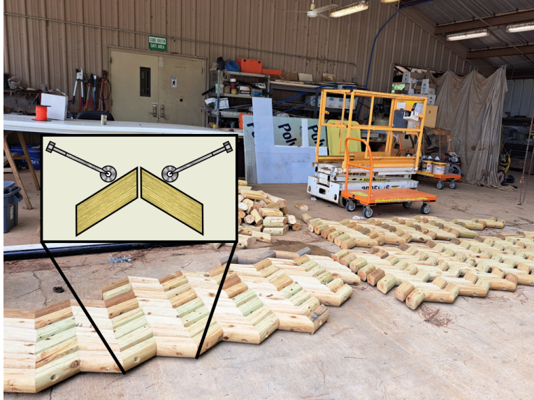
Figure 3.5.1 Climbing aid segments were pre-fabricated before installation
