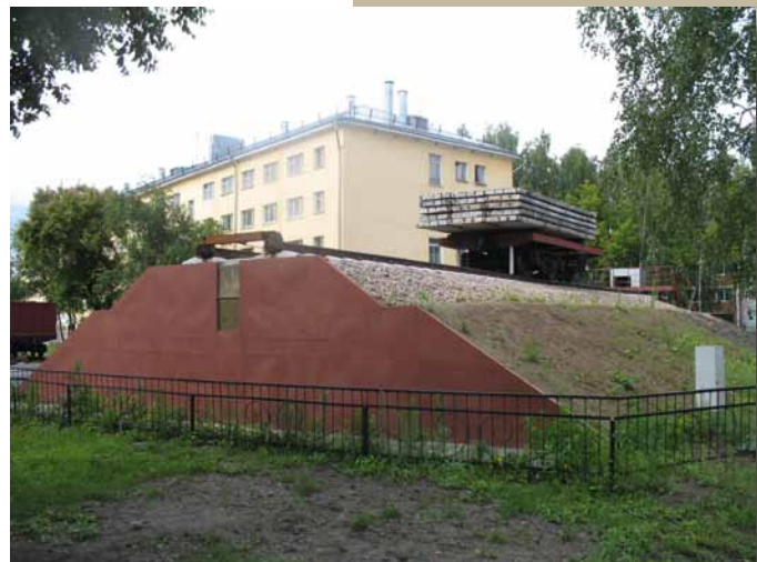
Railway embankment constructed for research purposes outside of the Siberian Transportation University in Novosibirsk, Russia.
