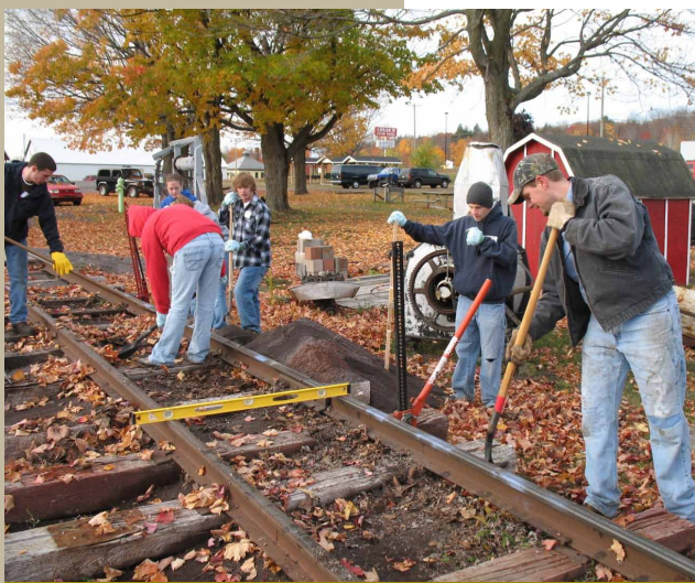
REAC Students leveling the Lake Linden Railway Museum track during "Make a Difference Day"
