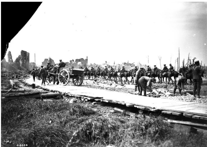
Canadian engineers building a corduroy road through a captured village during the advance, east of Arras in September 1918. [LAC Item ID 3405430]
