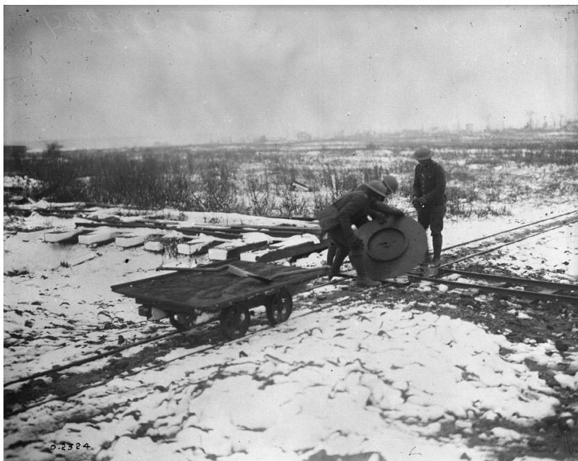
Canadian Railway Troops repairing a railway turn-table near Lens in December 1917. [LAC Item ID 3405545]
