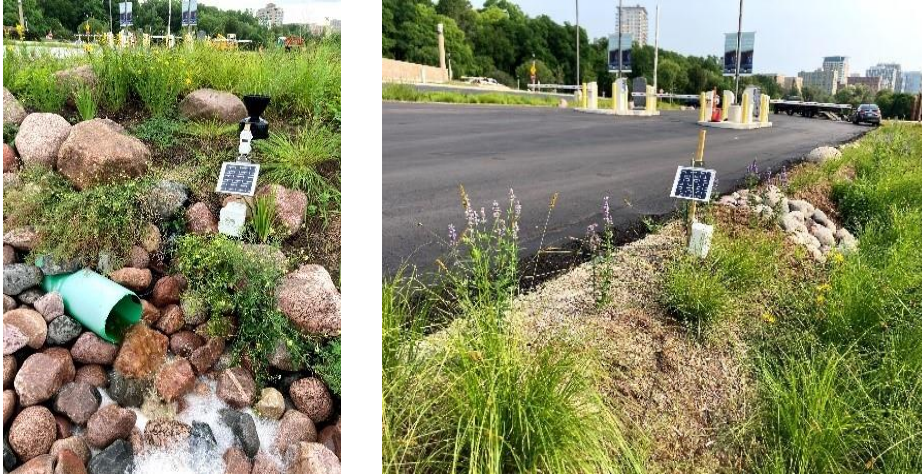
Figure 5-2. Bioswale 2 outfall into riprap channel, rain gage, and data logger (left); data logger in bioswale 2 that measures the discharge from the permeable paver and bioswale 1 underdrains (right).
