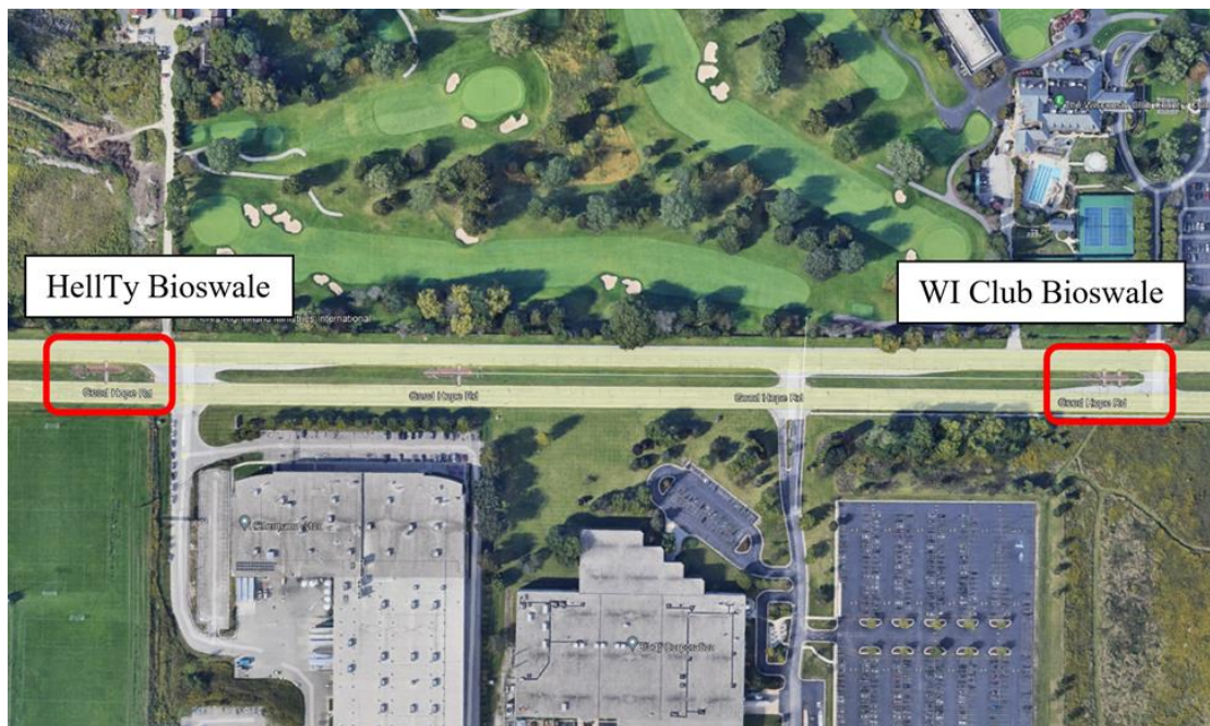
Figure A 4-5. Locations of the bioswales (HellTy Bioswale at the entrance to Hellermann Tython headquarters; WI Club Bioswale at the entrance to Wisconsin Club county club).
