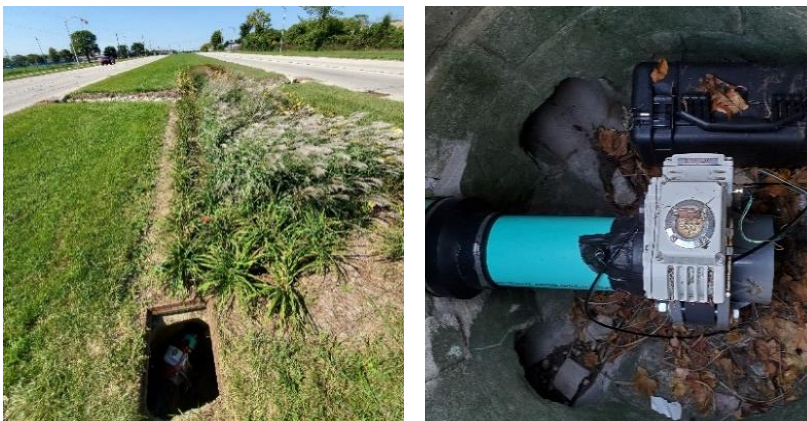
Figure A 4-7. The image on the left shows the HellTy bioswale with the overflow grate open and the active control visible; the image on the right shows the real-time control attached to the underdrain of the HellTy bioswale.
