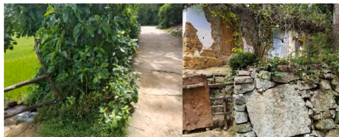
Fig. 1. Live fencing using pawatta ( adhatoda vasica ) plant and retaining walls. Source: Author.
