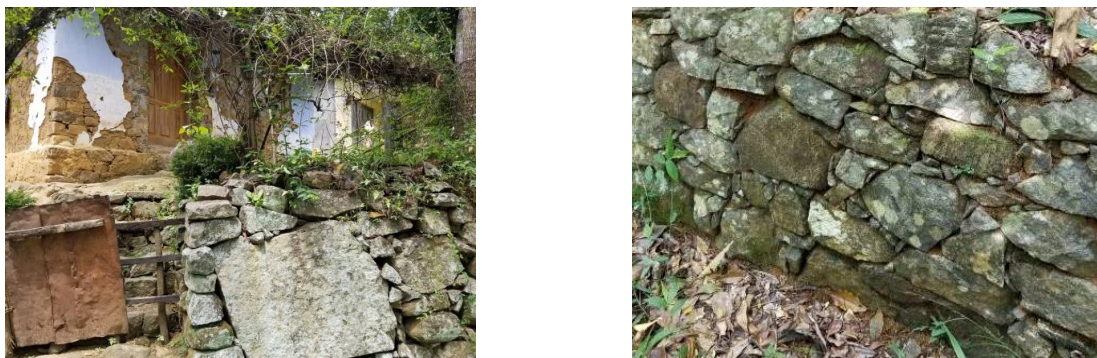
Fig. 7. Retaining Walls. Source: Author.
