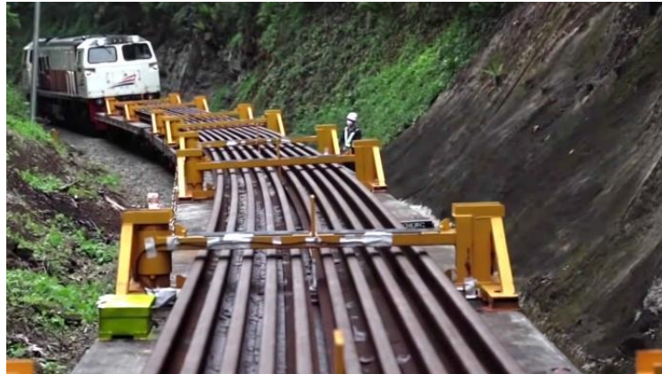
Figure 12 On-track test of long rail transport through a small-radius curve.
