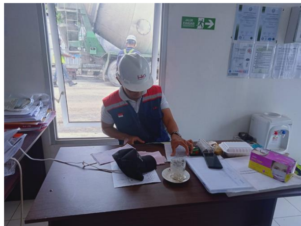
Gambar 2. 18 Pengecekan Docket Kedatangan Truck Mixer
