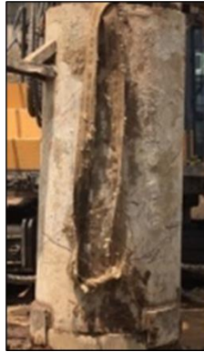
Gambar 2. 7 Casing Temporary
