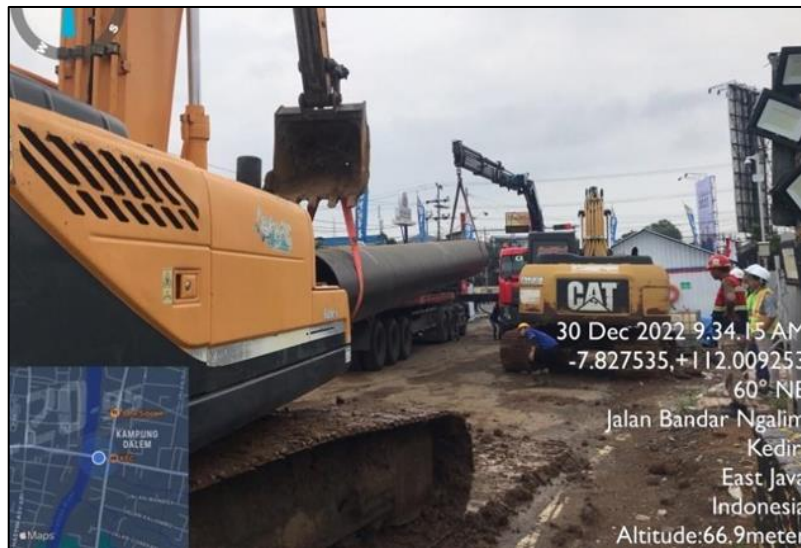
Gambar 2. 14 Mobilisasi Casing Permanent
