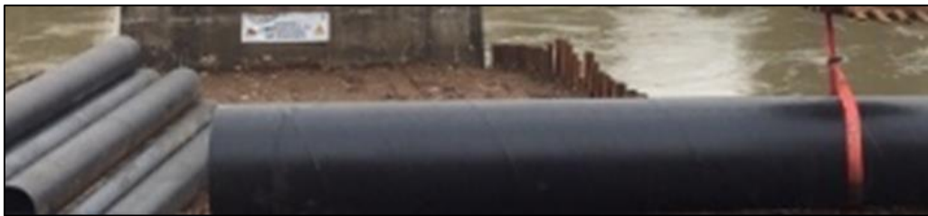
Gambar 2. 8 Casing Permanent
