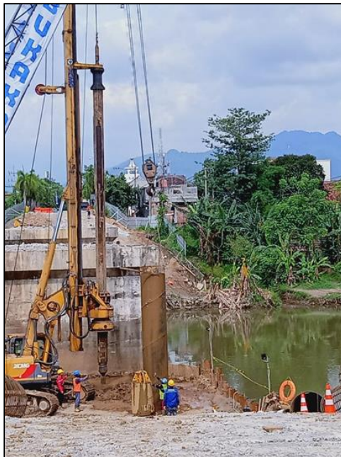
Gambar 3. 3 Pencabutan Casing Permanent P1.8
