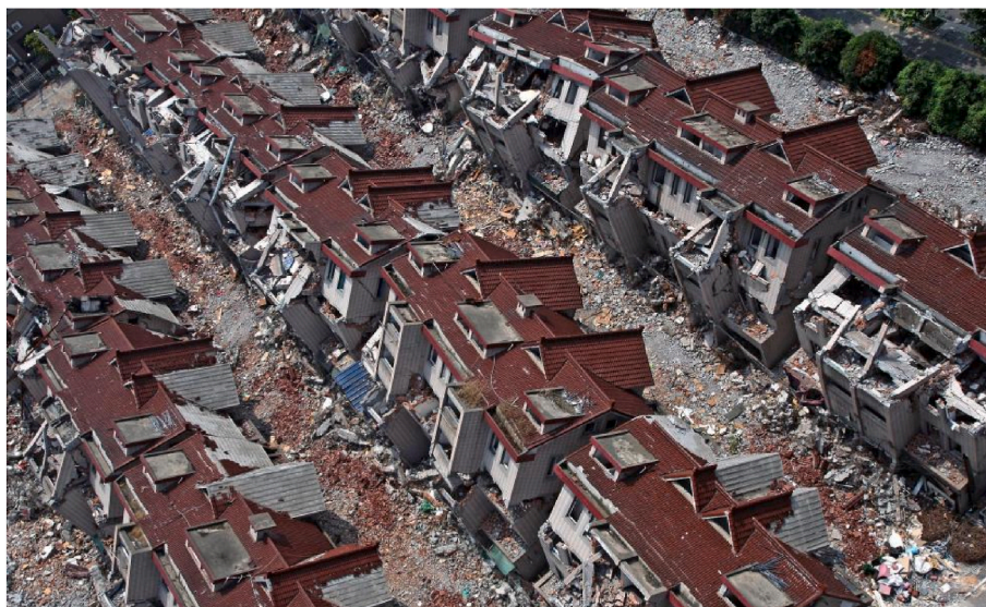
Fig. 1. Example of blind large-scale demolition in urban regeneration practices. (Source: Photo from Visual China Group, 2017)
