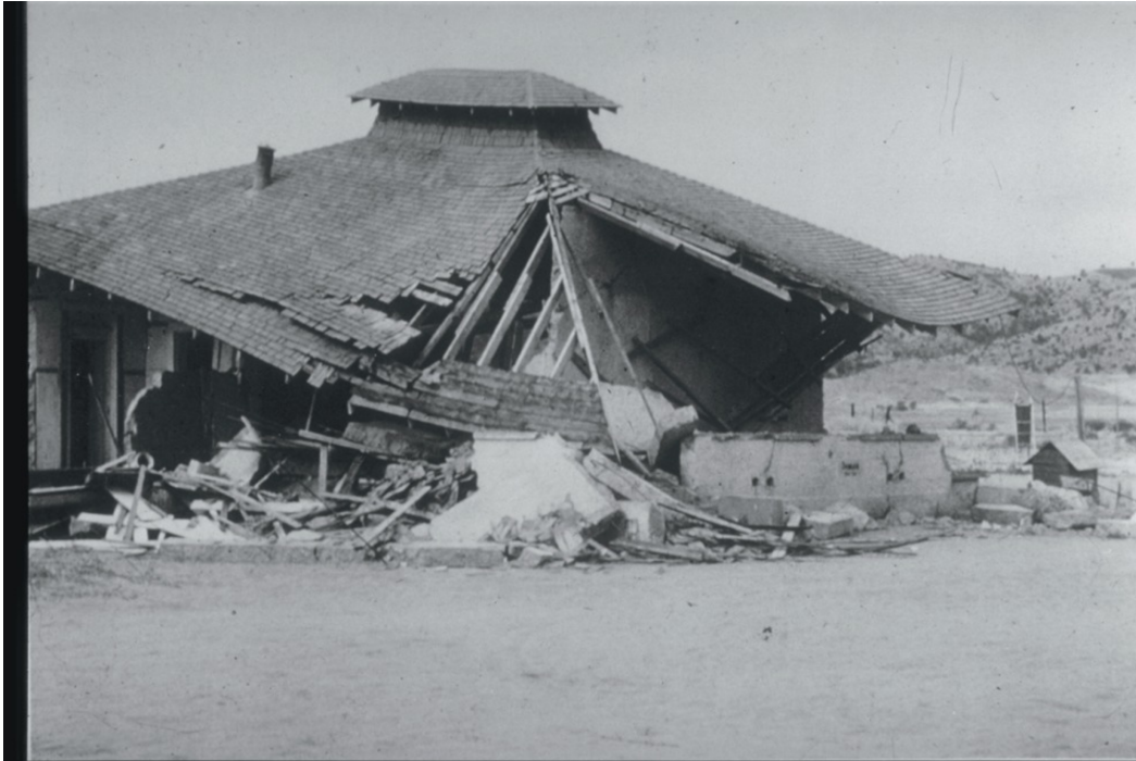
Fig. 10 Collapse of school building in Kern County, California from the 1933 Long Beach earthquake
