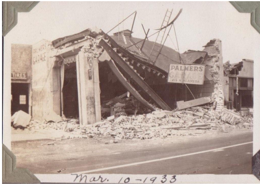
Fig. 8 Destruction of building by the Long Beach earthquake of 10 March 1933 (photo; U.S. Geological Survey)
