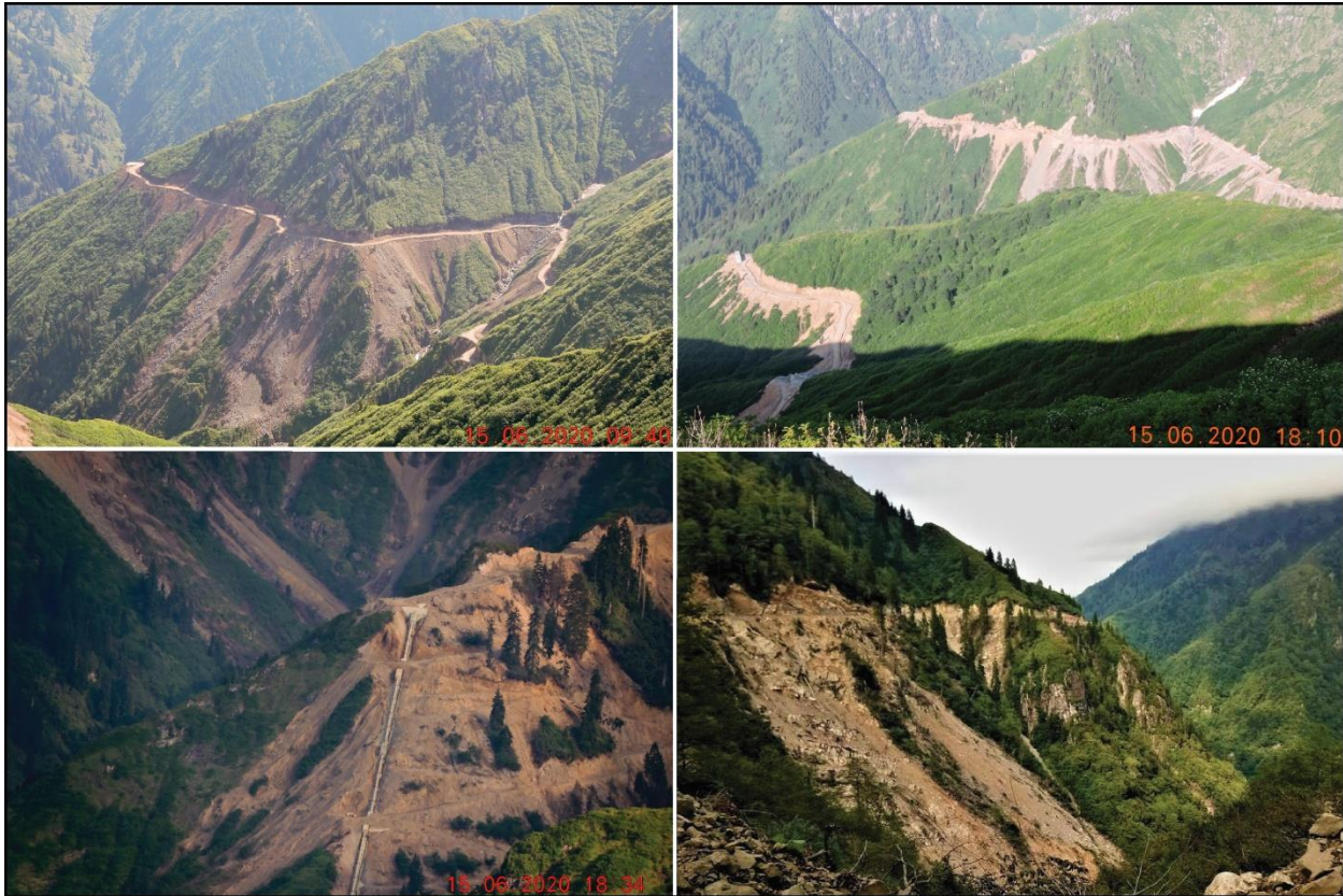
233 234 Figure 5. Photos showing the mass movements on hillslopes associated with road constructions 235 of HEPP . The photos were taken on 15 th June 2020 (Photographs courtesy of Hasan Sıtkı 236 Özkazanç).
