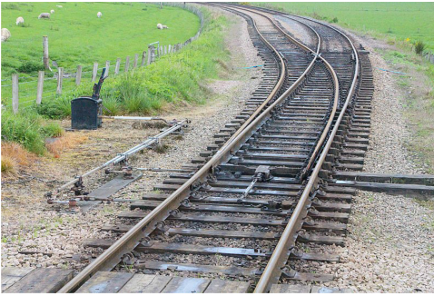
Fig. 2. Point at Broomhill station, Scotland [45].
