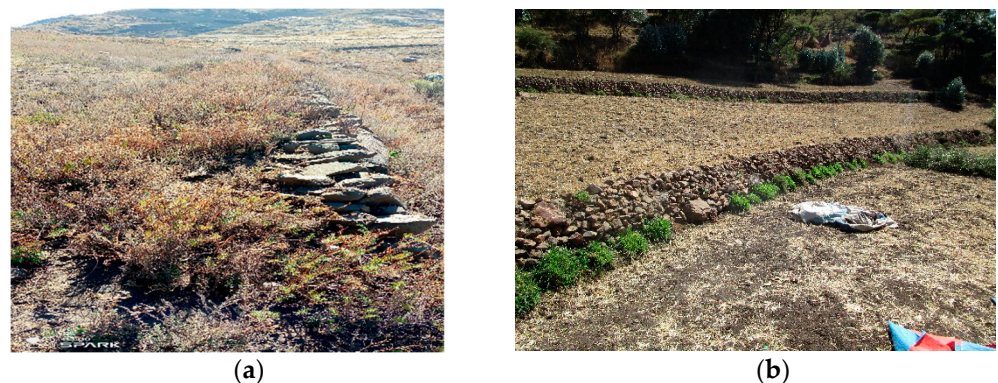
Figure 12. (a) Stone-faced bund covered with unpalatable plant species; and (b) broken and unmaintained bund on-farm plot.
